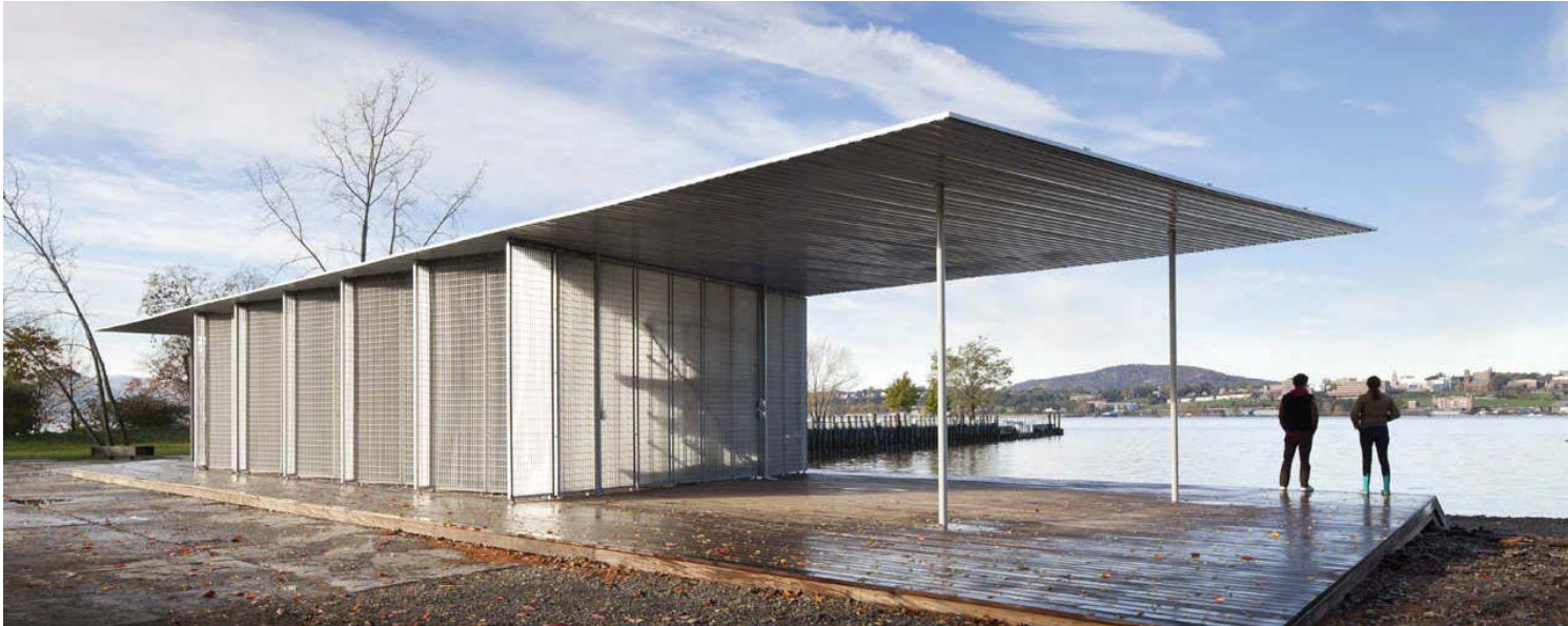
BEACON, NY | CORRUGATED ROOF SET ON STEEL COLUMNS
