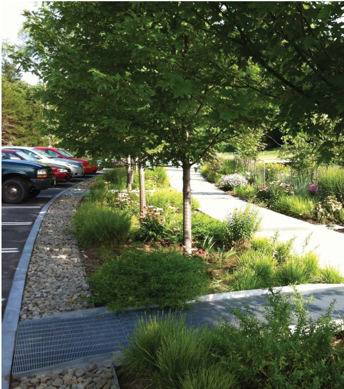
STONE FILTER BETWEEN RAIN GARDEN AND COMPOST FACILITY
