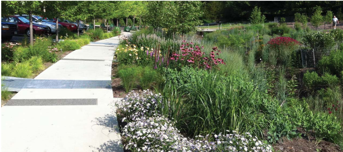
BIOSWALE, CORNELL, NY | BIOSWALE GARDEN WITH 1 ACRE COLLECTION AREA
